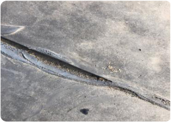
Figure 2: A seam patch on the roof had lifted.
