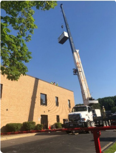
Figure 5: New HVAC unit being lifted to the roof
