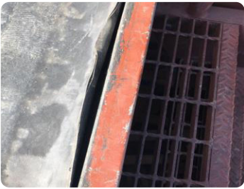
Figure 1: The roof's EPDM liner was loose around roof hatch.
