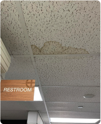
Figure 3: Water leakage was causing ceiling damage.
