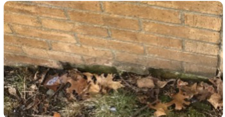
Figure 7: Decayed brick near the soil line was allowing water leakage into the ECC classrooms.
