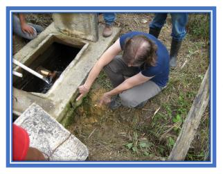
As you can see, there are many leaks. There are leaks in the collection tank, the pipes and the distribution tanks. The current water system was built in the 1980's and 1990's, designed for a maximum of fifty families.
